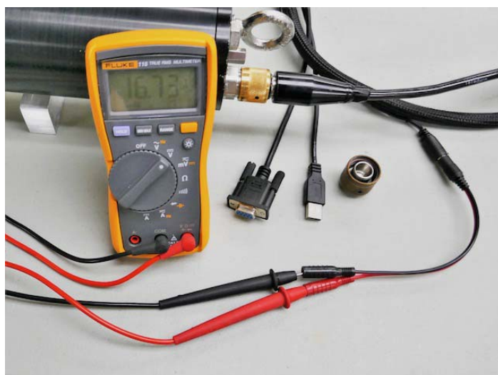
Figure 33: Connecting banana jack cable to deck cable and measuring the battery voltage
